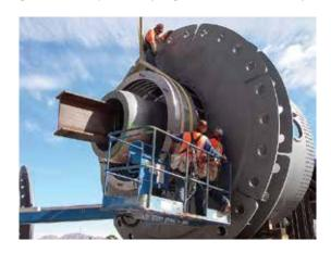
On the fabled Las Vegas Strip in the US, the High Roller ferris wheel contains two of the largest SRBs ever produced by SKF, each weighing in at 8.8 tonnes! SKF spherical roller bearings can be found in many applications, including some where you might not expect them. A good example is the Bahrain World Trade Center, where three tower wind turbines, each 29 metres in diameter, are architecturally installed
