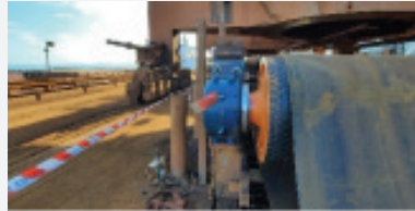
— P6: Installation of critical pulley with SAPO® Seals
